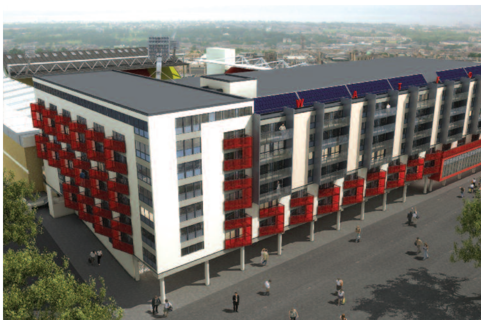
What the finished affordable homes at Watford stadium will look like
