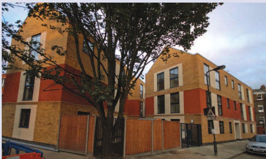
Recently finished Hemstall Corner, Camden.
